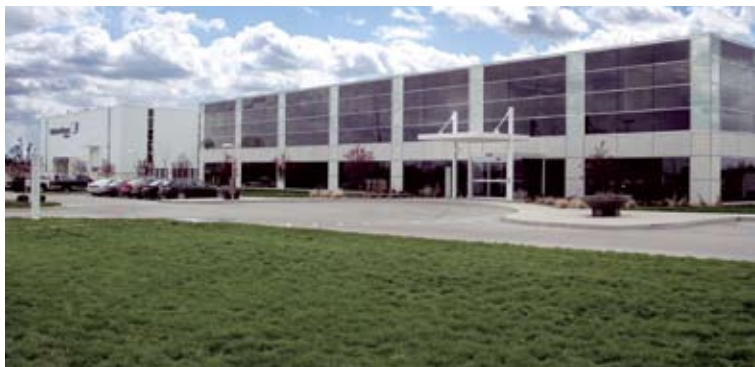
Magmeter manufacturing facility and calibration lab in Indiana
